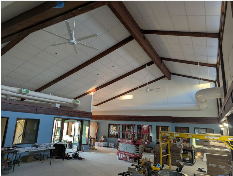
View with all the main office tiles and ceiling fans installed
