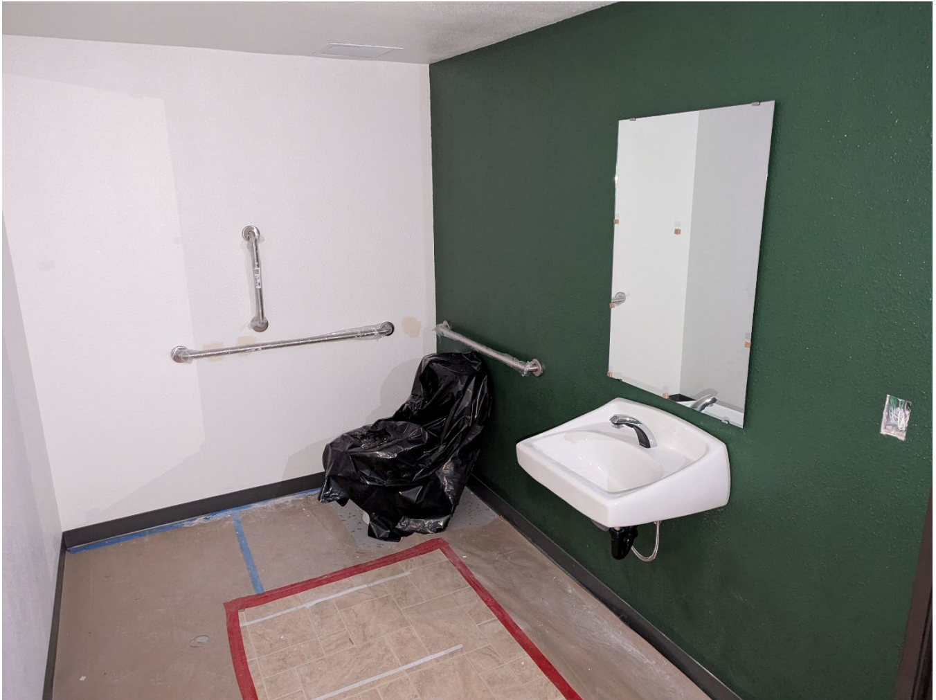
One of the main restrooms, still in need of some fixtures and lighting. Paper and scrap flooring installed for new flooring protection. All restrooms now meet ADA requirements.
