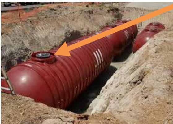
**Single Point** – If your facility has a single point Stage I system the tank would look similar to this one. One opening in the tank allows for both vapor return and liquid filling. Ensure the gasket seal is in good condition, the cap fits snugly and creates a good seal, and all spill containment buckets are free of liquid and debris.
