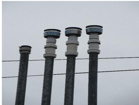
This picture shows three PV valves, one for each gasoline tank on site, and one open atmospheric vent (left) piped to the diesel tank. Note that one PV valve is acceptable for multiple gasoline tanks if the piping is manifolded together.
