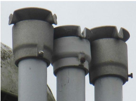
Open atmospheric vents (not PV valves). These open vents are always okay for diesel tanks. These vents are only allowed for gasoline tanks if your facility gasoline throughput has been below the threshold described in your permit for Stage I equipment.
