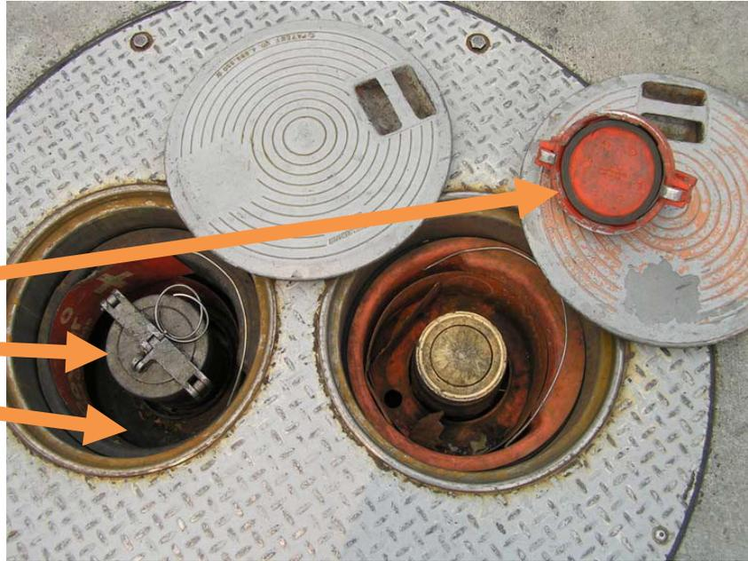
**Poppet Valve AKA Dry Break (Dual point)** – Does the spring movement open and then return to a closed/sealed position when depressed if you have it?
