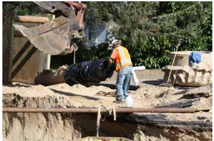
*LRAPA’s enforcement and compliance staff respond to complaints and perform inspections. The top photo was taken by staff at a residence where illegal burning occurred. The bottom photo shows work being done on a sewer project where old pipe containing asbestos had to be properly removed and bagged for disposal. Staff conducted regular inspections to ensure compliance with LRAPA rules.*
